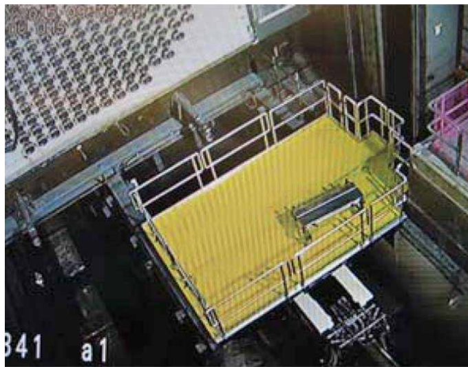
Figure 3: Platform in use (1/2 deployed)
