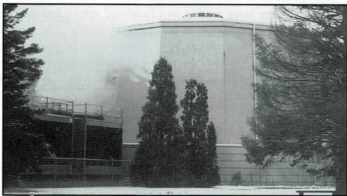
A recent view of the MNR containment building and new cooling towers (at left).
