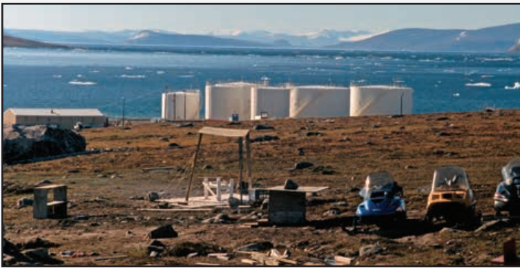
Fuel storage tanks, Clyde River, Nunavut.
