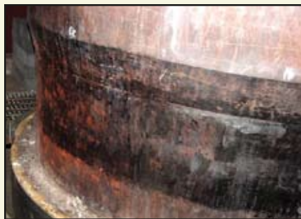
▲ Figure 5-9: Steam Generator to Steam Drum Connection
