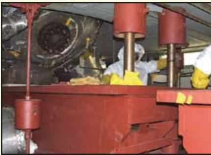
▲ Figure 5-12: Vault Showing Limited Head Room between Top of Support (Trapeze) & Vault Ceiling
