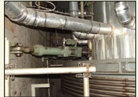
▲ Figure 5-2: Boiler Room, top of the Containments Seal Assembly & Seismic Restraint
