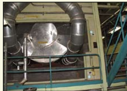
▲ Figure 5-10: Steam Drum Face Showing Cooling Ducts
