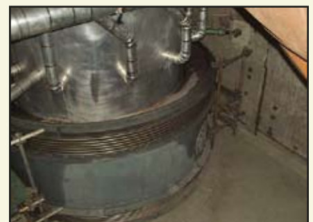
▲ Figure 5-4: View Inside Boiler Room Above Vault Showing Containment Expansion Joint & Blow Down Lines
