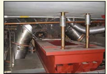
▲ Figure 5-14: Vault PHT Inlet & Supporting (Trapeze) Arrangement
