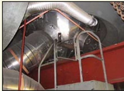
▲ Figure 5-13: Vault PHT Piping & Support Arrangement
