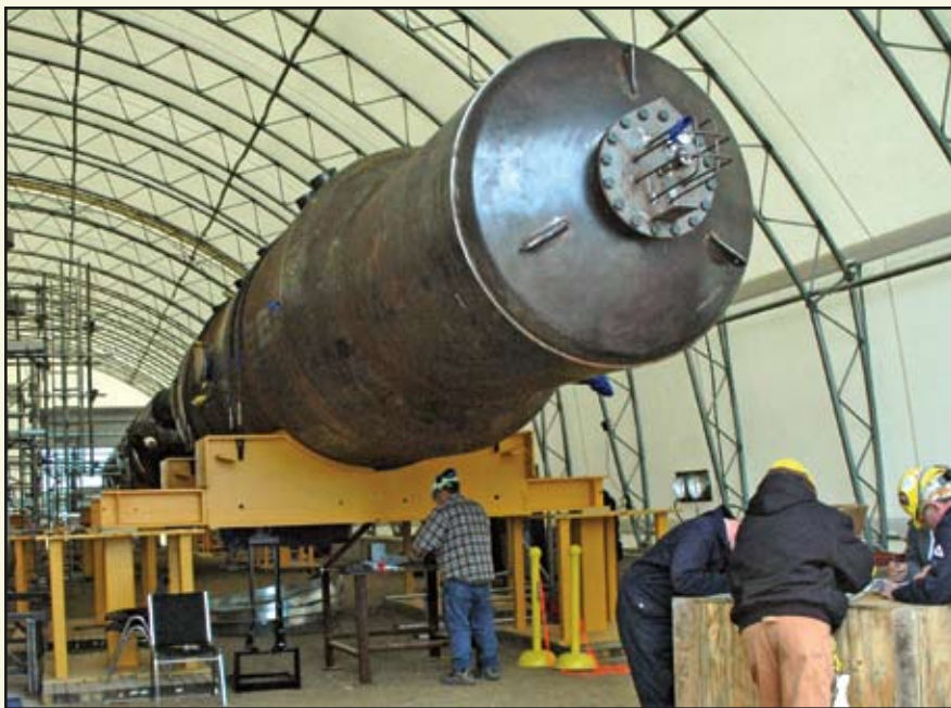
To give an appreciation of the size of the steam generators, this view shows tradespeople from Comstock Canada working in a temporary storage building on new steam generators for Unit 2. Comstock is a subcontractor on SNC-Lavalin Nuclear's steam generator replacement team.
