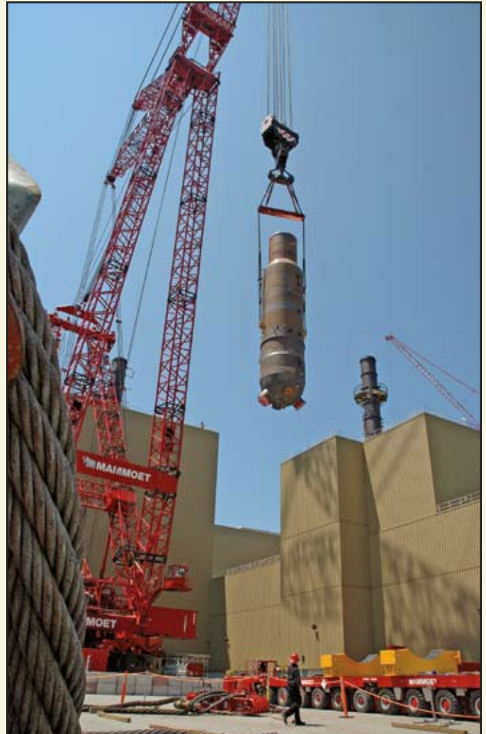
A view of the first new steam generator being lifted into place into unit 2 by the huge Mammoet crane on June 13, 2007.
