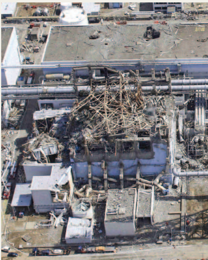
Figure 6: Massive damage at Unit 3 following the hydrogen explosion on March 14.
