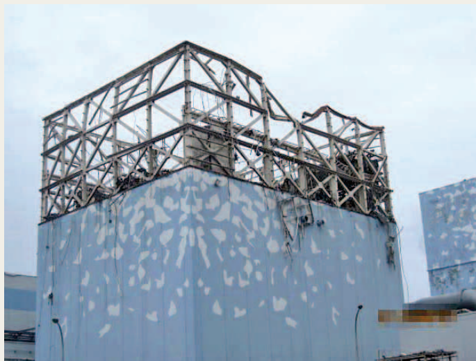
Figure 5: Result of the first hydrogen explosion in Unit 1 on March 12.
