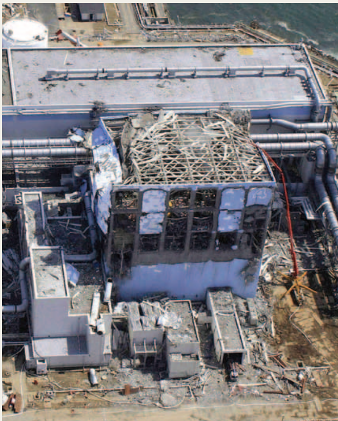
Figure 4: A reverse flow check valve could have prevented the explosion in Unit 4.
