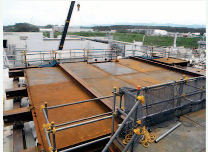
The steel platform in place over the used fuel pool of unit 4 (Image: Tepco)
