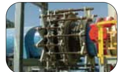
Inline Pressure Balanced Rubber Expansion Joint
