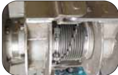
Dousing System Hinged Expansion Joint
