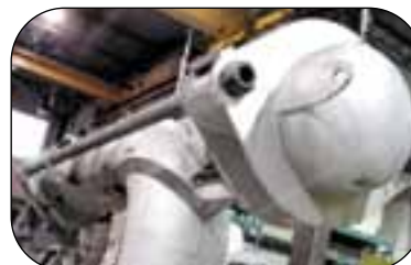
Main Steam Crossover Expansion Joint
