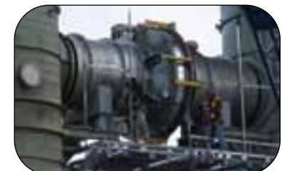
Inline Pressure Balanced Expansion Joint
