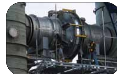
Inline Pressure Balanced Expansion Joint
