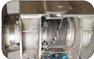
Dousing System Hinged Expansion Joint
