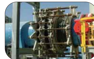
Inline Pressure Balanced Rubber Expansion Joint
