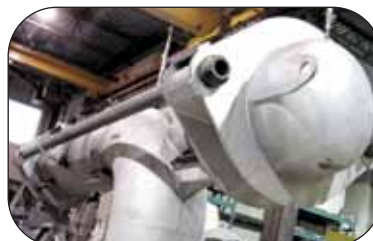
Main Steam Crossover Expansion Joint
