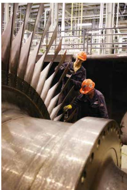
Lower pressure turbine blades undergoing inspection during routine maintenance outage. (Photo courtesy of OPG)
