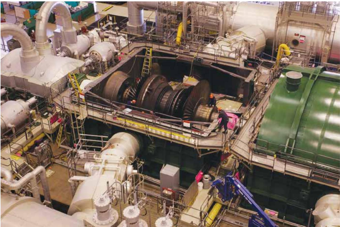
Unit 3 low pressure turbine open for inspection during routine maintenance outage. (Photo courtesy of OPG)
