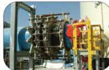
In-line pressure balanced rubber expansion joints
