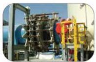
In-line pressure balanced rubber expansion joints
