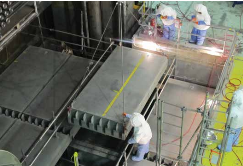
Hoisting East side Unit 1 bulkhead panel. (Bruce Power photo)
