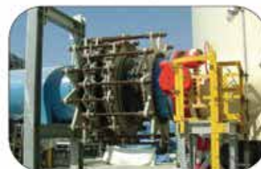
In-line pressure balanced rubber expansion joints
