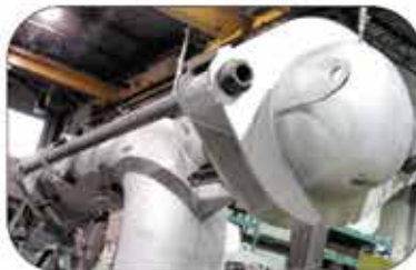
Pressure balanced crossover expansion joints
