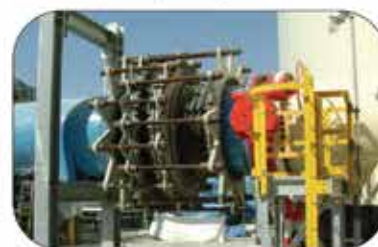
In-line pressure balanced rubber expansion joints
