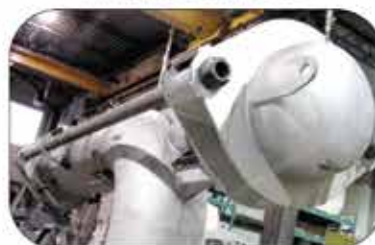
Pressure balanced crossover expansion joints
