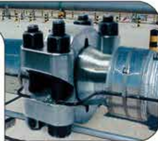
2500 psi steam piping system with Thorloc 316SS 4 inch connector
