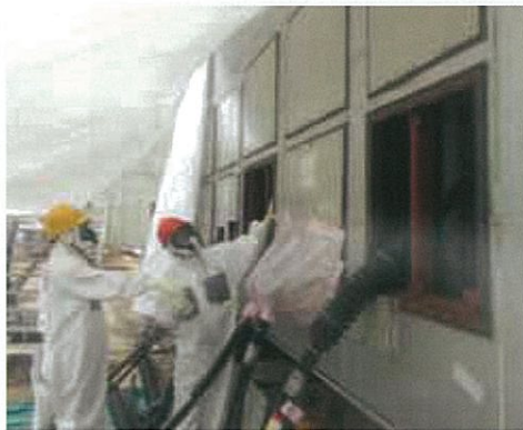
Inspection of Units 3-4 temporary M/C.
