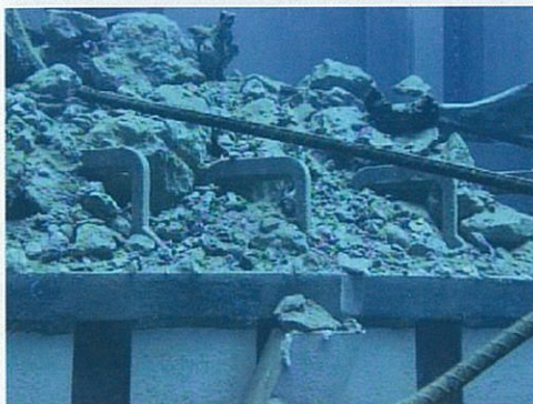
Lower photo: close up of sediment on the fuel rack
