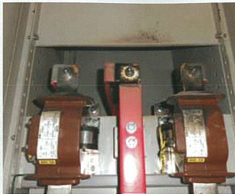
Soot found on the instrument current transformer.
