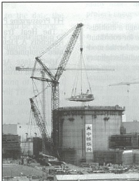
Figure 2 – Lowering of a Dousing System Module Through "Open Top at Qinshan
