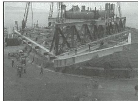
Figure 3 – Positioning of a Dousing System Module at Qinshan
