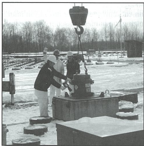
Figure 3. High-activity waste being transferred from a shipping flask into standpipe storage. Adjacent standpipes are covered with resusable shielding plugs.
