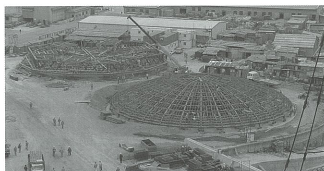
Figure 10: Dousing Steel and Lower Dome Formwork Assembly Area at Site (Unit 2)
